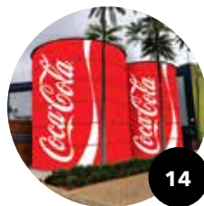
WATER TANK BRANDING
